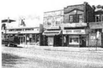
Retail Frontages on 3600 Block of Georgia Avenue
