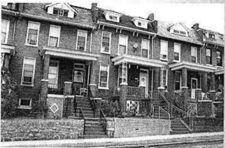
Quincy Street Row Houses
