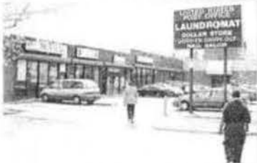
Retail Center at 3300 Block of Georgia Avenue
