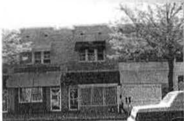
Retail Frontages on 3200 Block of Georgia Avenue
